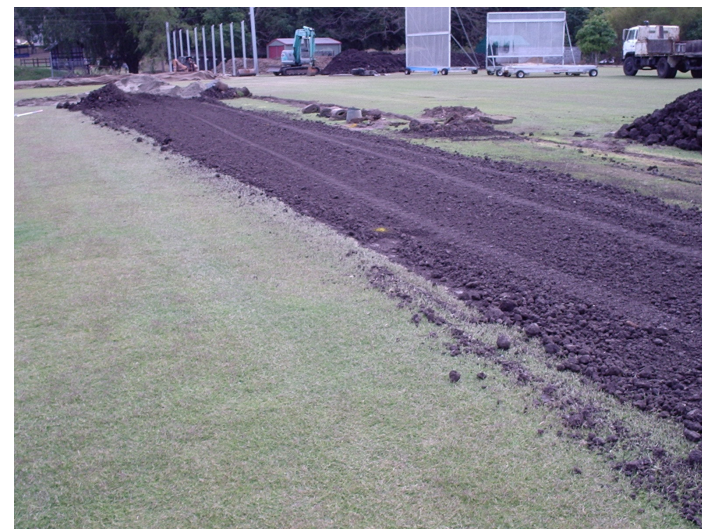
Figure 14 - Spreading of black soil
