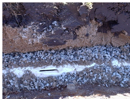
Figure 10: Drainage slotted 90ml PVC or Ag Pipe
