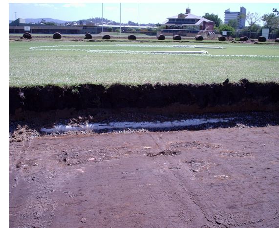
Figure 5: - Wicket depth and drainage
