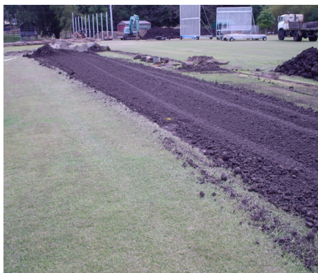
Figure 1: Spreading and levelling wicket soil
