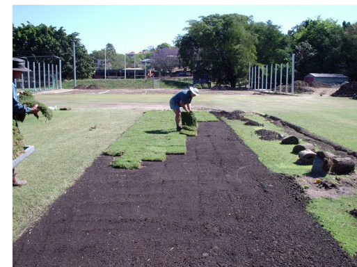
Figure 6: - Laying full turf on new wicket.
