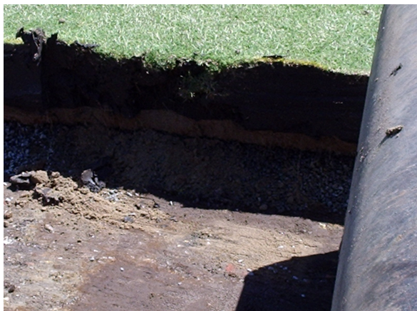
Figure 4 - Wicket depth with underlays
