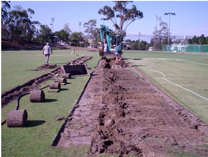
Figure 15 - Excavating wicket site
